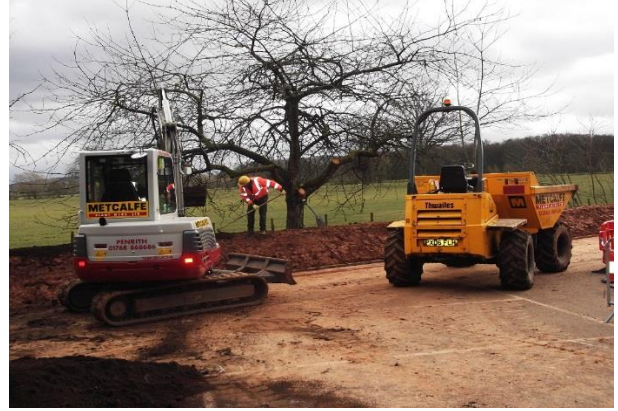
Construction of clay and soil earth bund
