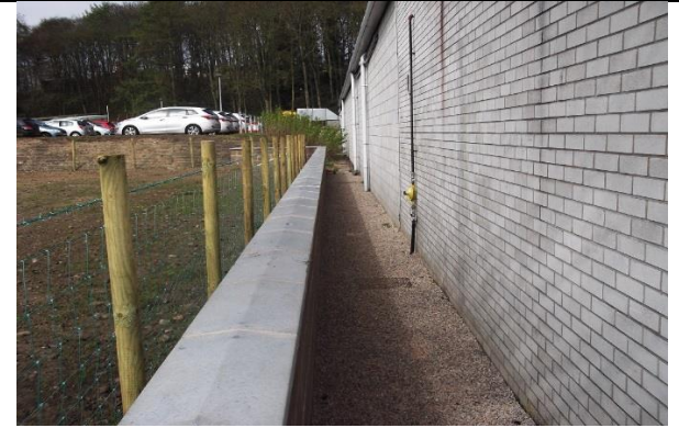
Pathway created after construction of flood wall
