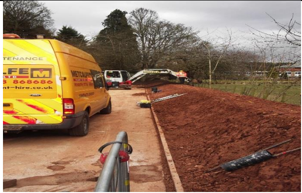
Earth bund landscaped prior to erection of lighting columns
