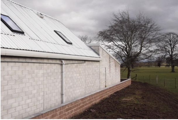
Flood wall constructed to southern end of firing range building
