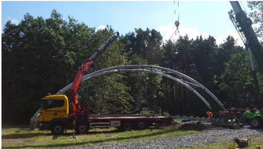
The bridge was fabricated off-site and delivered in kit form. It was built and lifted in using a crane and hi-ab.
