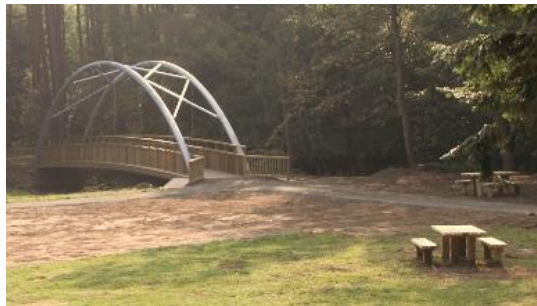
The bridge was fabricated off-site and delivered in kit form. It was built and lifted in using a crane and hi-ab.
