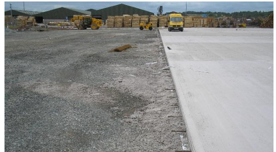
The finished slab area was 8500m 2 , and used 1700m 3 of concrete.
