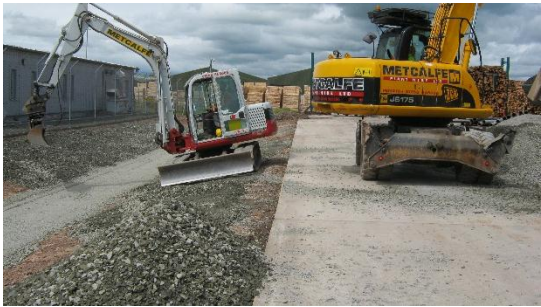
The existing swale was re-graded and trimmed with sub-base.
