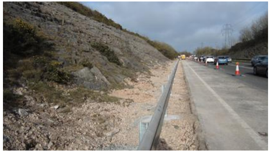
A section of crash barrier that has been replaced.
