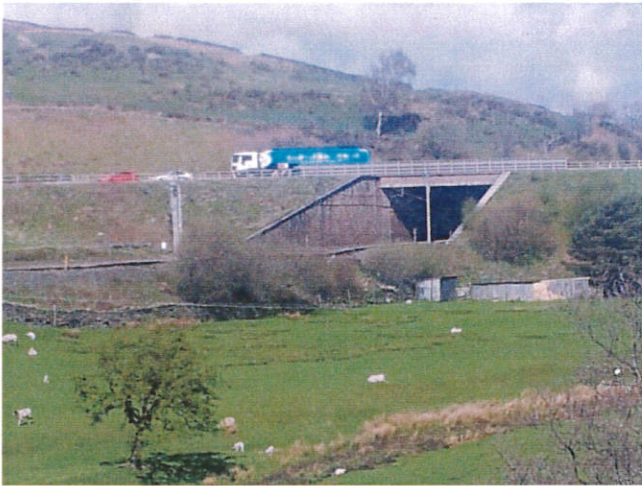
View of the M6 Loups Fell bridge prior to works being commenced.
