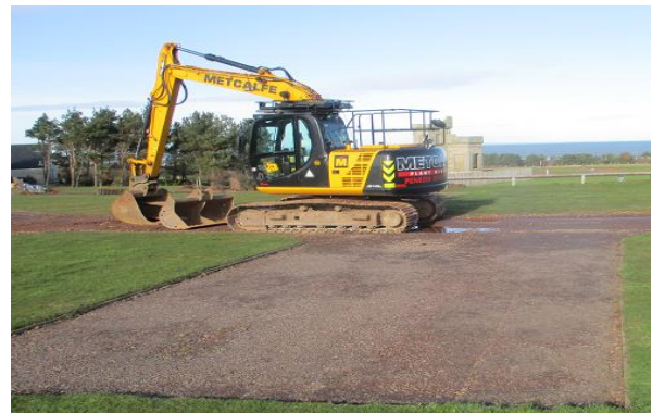
Large MPH JCB excavator required on existing hard ground
