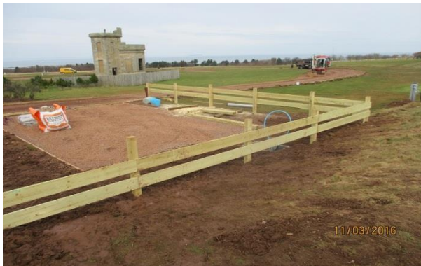
Site Manager Pitch with timber fencing
