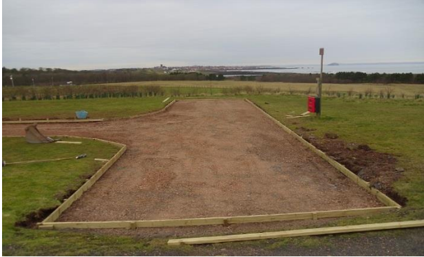
Subbase and timber edgings to site roads.
