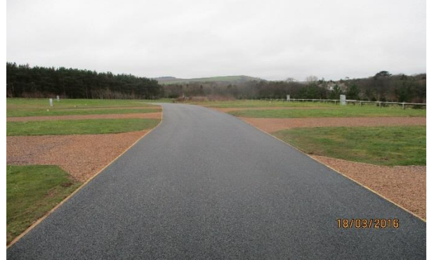
Tarmac to site road and completed pitches
