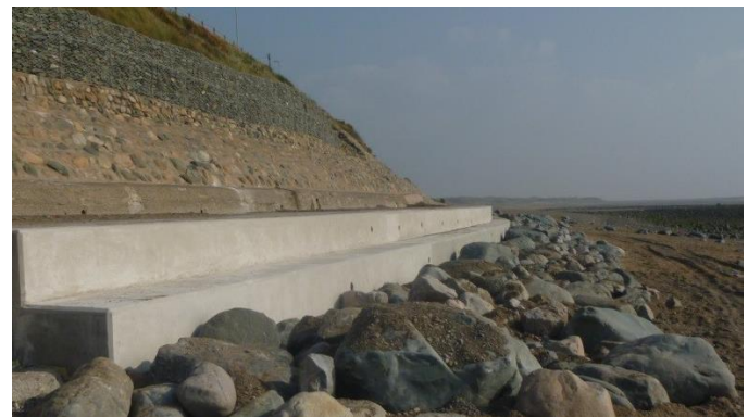
The finished length of wall with the rock armour in place.
