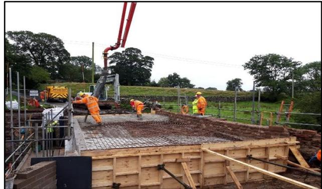
New concrete saddle to the existing stone arch barrel
